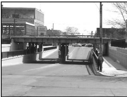
CPR low-profile bridge at Dovercourt Rd.
