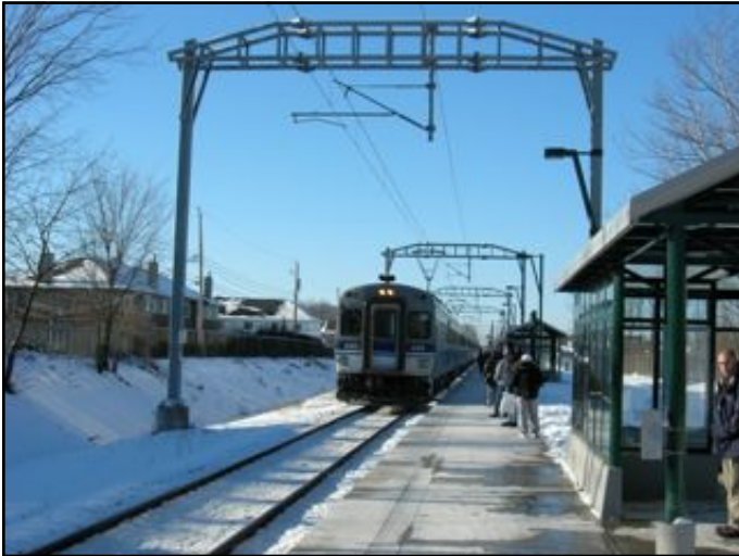
Montreal's Electrified Two-Mountains line (AMT) using multiple unit electric trains built by Bombardier. Photo by Justin Bur.
